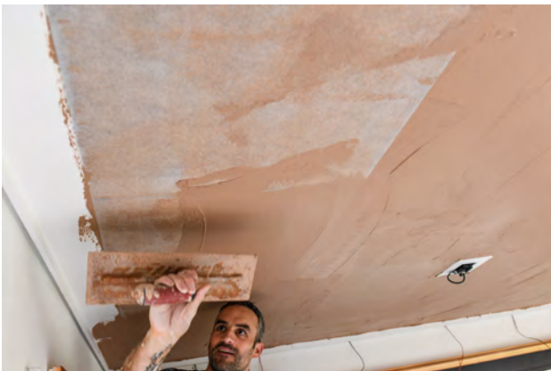
The plaster will start to come through the fleece and seal the fleece into the plaster, continue plastering until a smooth finish is achieved before starting the next heating fleece placement
