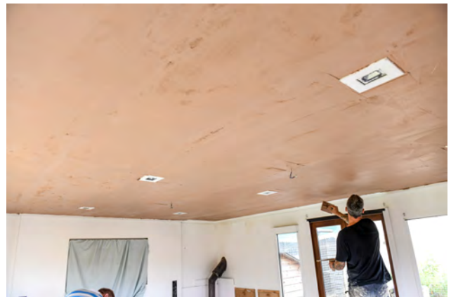
If using a plasterboard adhesive this must be dry before the final plastering finish can be applied. If using a wet mix of multi-finish the second final plaster coat
