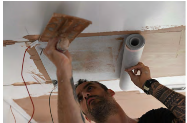
start to unroll the heat panel approx 12-18" at a time, using a nylon trowel, firmly start to trowel in the direction of the material roll
